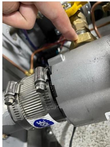
2. Loosen the two screws on the air intake coupling below.
