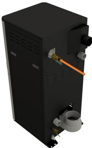
The gas pipe connection to the Valiant FT can be found at the rear of the unit (Figure 15).
