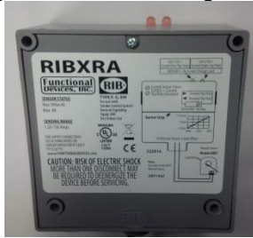
Figure 20: Flow Proving Device
